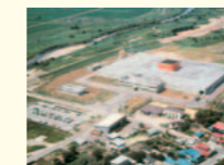
Takahata (Yamagata) Plant completed (1974)
