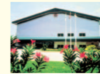
Start of operations at Siam Okamura Steel Co., Ltd. (Thailand) (1988)
