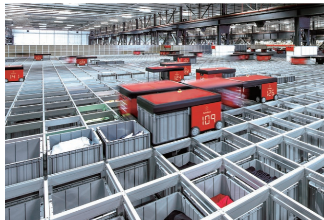
Robot storage systems
