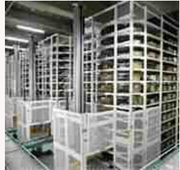
Automated storage system
